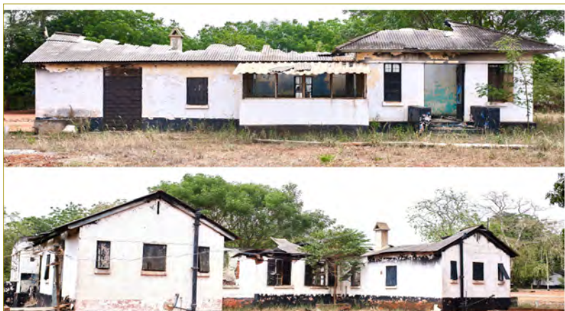
Burnt Out Structure: Behind Clark House
